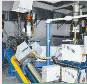
550 kV Maillefer HVCV Insulate Line
